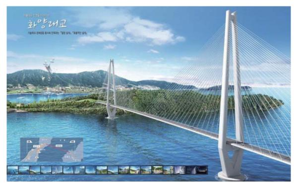
화양대교(화양-적금 2공구) Scope:Length = 854.0m, Main Tower Height= 170.7m, Interval = 500.0m
