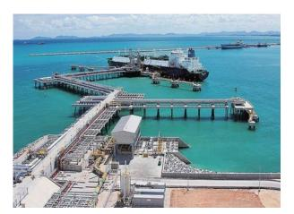
PTT LNG receiving terminal project (태국) - W/ P :1set, BD:3set, MD : 6set, Trestle : 250m - Design Vessel : 266,000m<sup>2</sup> Carrier
